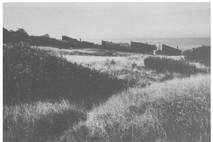
Fig. 3. Sea Ranch. Landscape and building form reflect the dominant wind patterns of the North California Coast. (Lawrence Halprin, Landscape Architect.)
